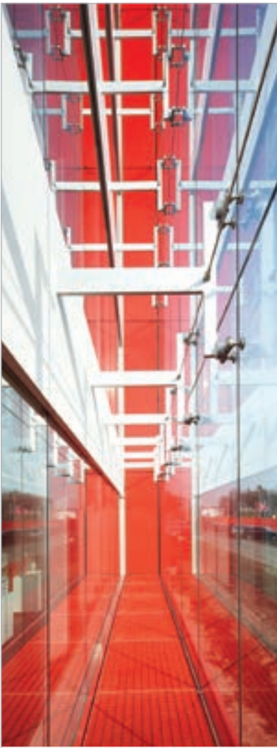
Hightech construction of the new Soudal building
